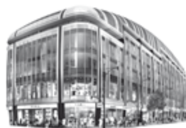
Park House, W1
